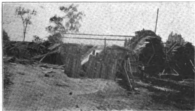
Form Work for Concrete Arches, Station 396.
