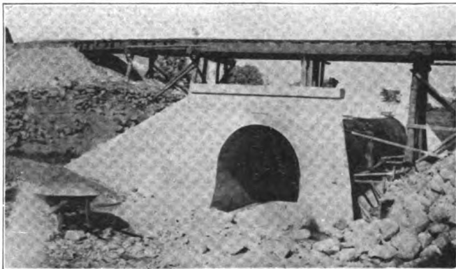
10 Foot Concrete Arch, Station 178+70.
