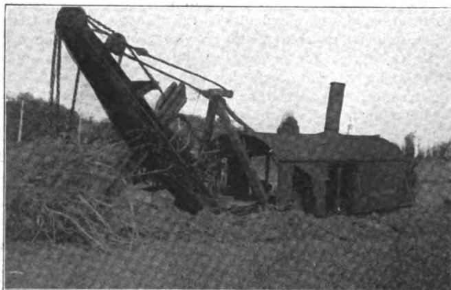
Bucyrus 97C Steam Shovel Starting Work at Blue Mound Cut.
